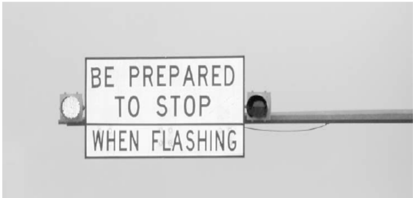
EXHIBIT V-5 Advance Warning Sign in Advance of a Signalized Intersection (Atlanta District, TxDOT)
