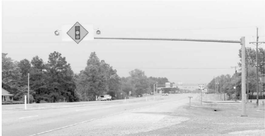
EXHIBIT V-4 Advance Warning Sign in Advance of a Signalized Intersection (Atlanta District, TxDOT)
