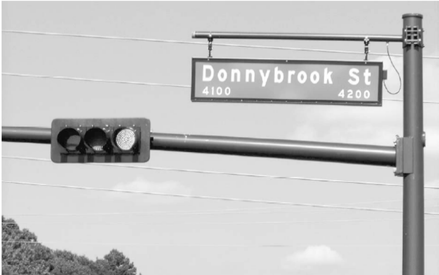
EXHIBIT V-9 Internally Lit Street Name Sign at Intersection (Atlanta District, TxDOT)
