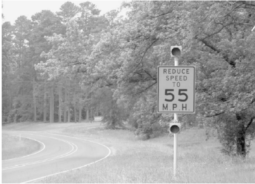
EXHIBIT V-6 Advance Warning Sign in Advance of a Horizontal Curve (Atlanta District, TxDOT)
